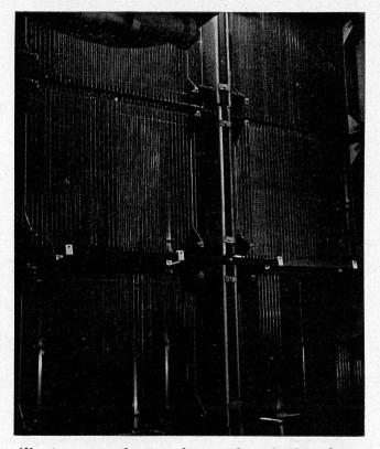
All air enters the greenhouses through this electric precipitator. Streaks of light, lower left, are sparks between plates, caused by insects being electrocuted.
