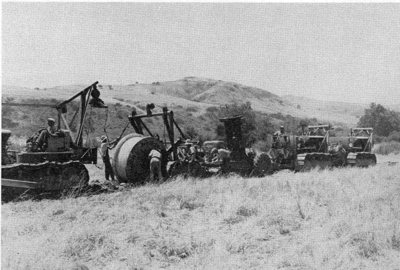
Preparing to load a new reel of cable among western hills. The gas tank on the side of the plow supplies pressure for the oil sprayer.
