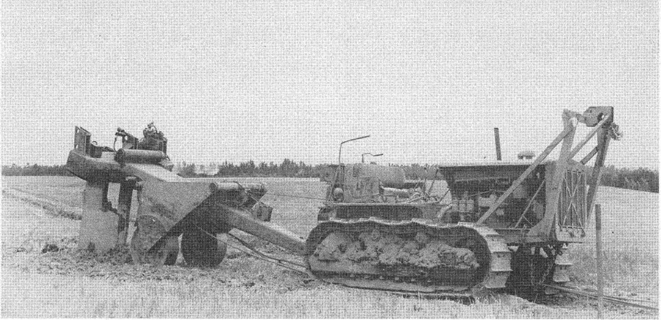
A special type of roofer plow used in opening a slot and later placing a cable six feet deep. The heavy steel ropes are attached to tractors outside the picture.
