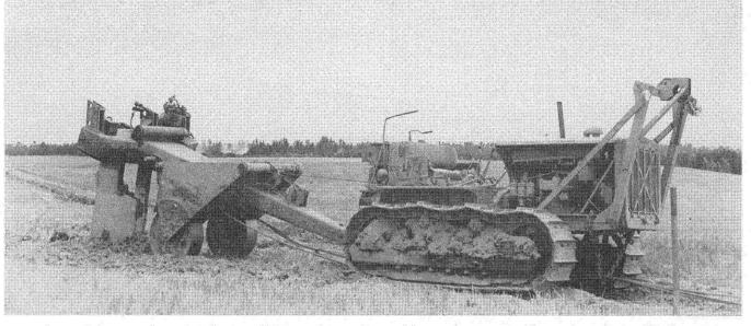
A special type of rooter plow used in opening a slot and later placing a cable six feet deep. The heavy steel ropes are attached to tractors outside the picture.
