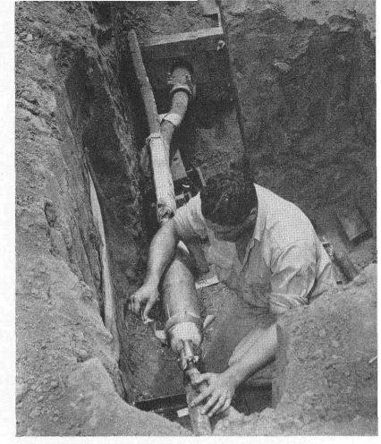
Splicer finishing a "wiped joint" over a splice. Cables bending away from the main cable are stubs to loading coil cases which are buried in their shipping boxes. The splice will be covered with a metal mesh and a protective covering before the pit is filled.
