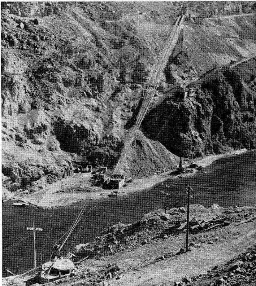
Figure 3. General layout of Guy F. Atkinson Cableway and Incline Hoist. (Note main cable around anchor in the foreground is three inches in diameter.) Courtesy U.S. Bureau of Reclamation, Boulder City, Nev.
