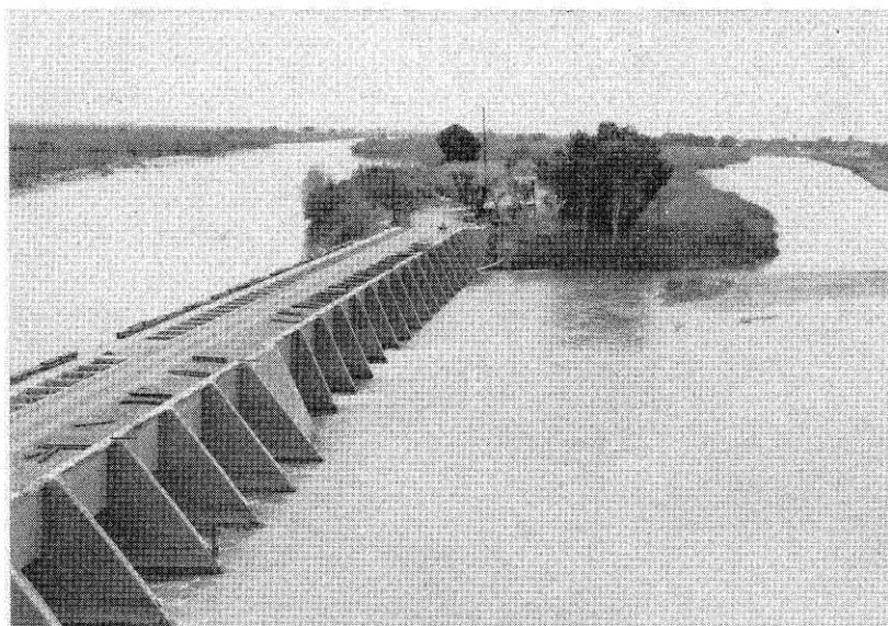
Plate 5. Rockwood Heading, showing the Colorado River to the left and the Alamo Canal to the right. Water is diverted to irrigated lands in Mexico. Formerly all Imperial Valley irrigation water passed through here.
