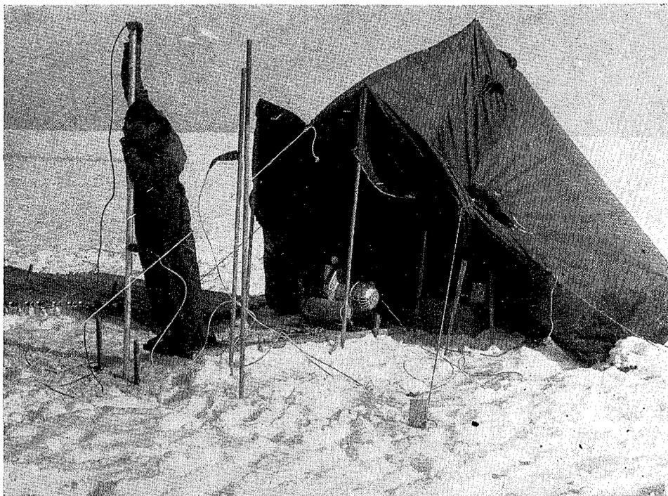
Boring a thousand-foot hole into ice by means of an electrically heated hot point.
