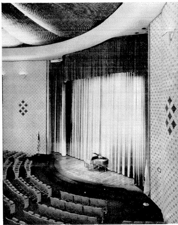
*The interior of the auditorium is dramatically decorated in red, white, and gold. The ceiling, made of anodized aluminum discs attached to fiberglass tape, gives the effect of a filigreed gold curtain.*
