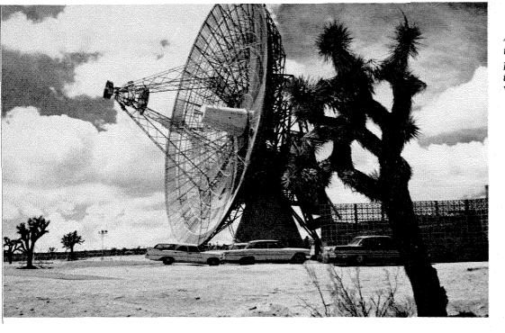
At JPL's Goldstone Tracking Station in the Mojave desert, this 85-foot parabolic dish is used for investigations of the surface features of Venus.
