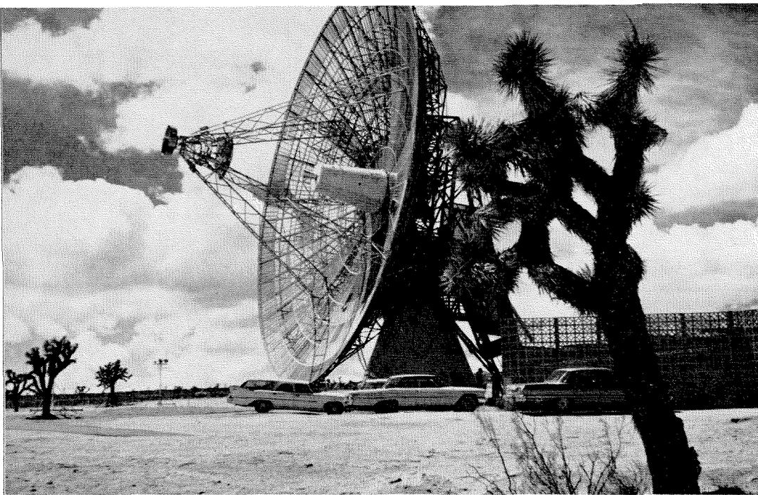
*At JPL's Goldstone Tracking Station in the Mojave desert, this 85-foot parabolic dish is used for investigations of the surface features of Venus.*
