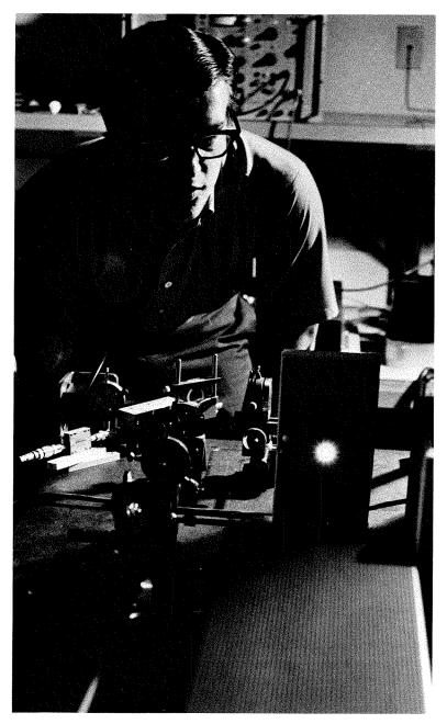
Research fellow Robert Menzies activates a highpowered carbon dioxide laser resembling the ones that will one day be used to detect pollution violators. The laser mechanism itself is contained in the long rectangular box at the lower right. The bright spot is the fire brick safety shield glowing white hot from the laser beam, which is invisible because it's in the infrared portion of the spectrum.
