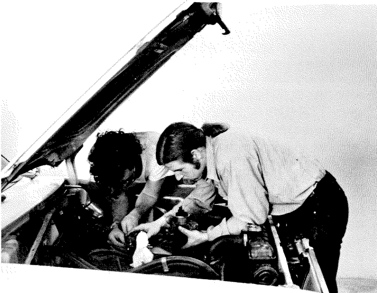
Gary Rubenstein and James Henry are converting Caltech's security car to the use of propane instead of gasoline. Because this car must idle or be driven at very low speeds a great deal of the time, use of propane should improve its efficiency as well as reduce emissions.
