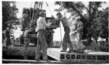
Swinging the assembled concrete beams into place to form the deck cover for the bridge. Beams are only 11%' deep.
