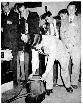
Visitor holds down metal ring against the force of an a.c. magnet in electrical engineering demonstration—
