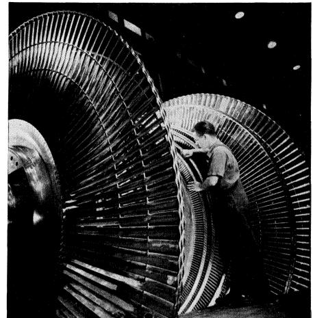
High temperatures and speeds raise tough design and production problems on giant steam turbine spindles like these.
