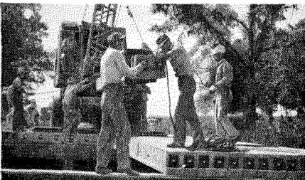
Swinging the assembled concrete beams into place to form the deck cover for the bridge. Beams are only  $1\frac{1}{8}$ " deep.
