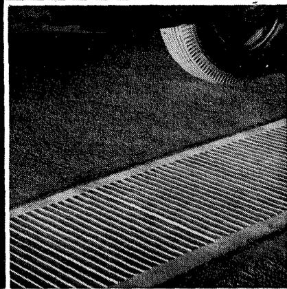
**ROAD SEPARATOR THAT TALKS.** Supplying reinforcing steel and cement for modern highways is one of the important jobs of United States Steel. Making highways safer is another one. This traffic lane marker, developed by Universal Atlas Cement, does double safety duty. Made of Atlas white cement, it is clearly visible at night. And its corrugated design (inset) actually causes it to sound a plainly-audible warning should you veer out of lane and your car tires ride on the corrugations.
