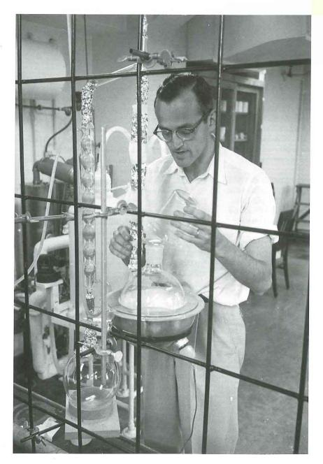
Patterson uses a distillation apparatus to purify reagents in his Caltech lab in 1957. He didn't trust the purity of commercial chemicals, so he redistilled them.
