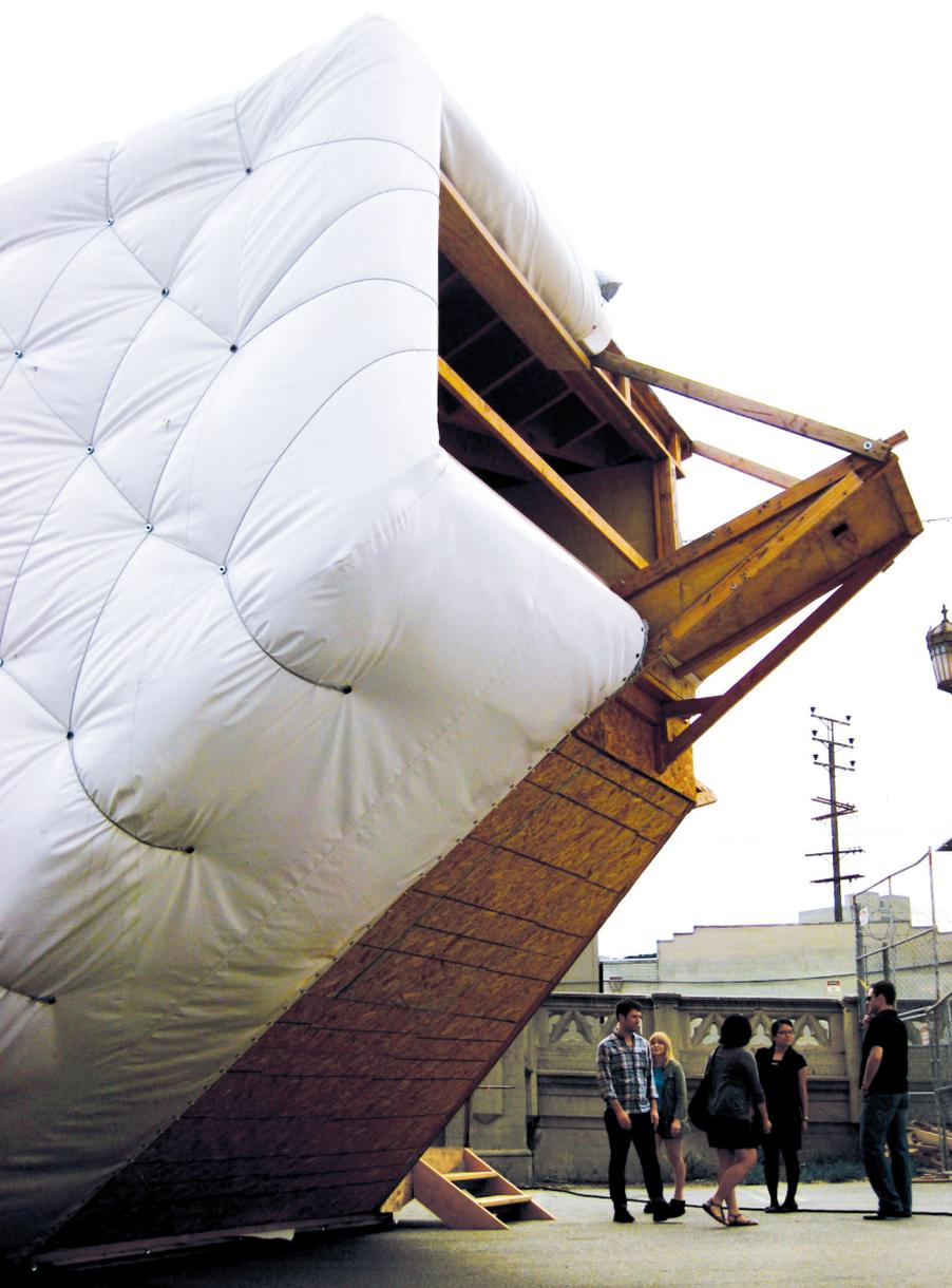
The full-sized mock-up of the SCI-Arc/Caltech Solar Decathlon house is partially covered in a soft, insulated "skin" of architectural vinyl.
