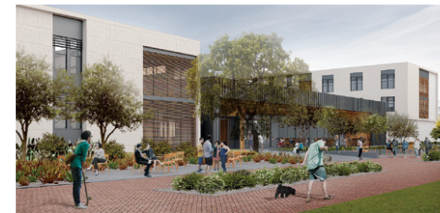
Work is well underway on the Bechtel Residence, Caltech’s newest undergraduate housing facility. A student committee and Student Affairs staff members are both currently exploring how to best use the 95,000-square-foot residence—named for Caltech life trustee Stephen D. Bechtel, Jr.—which is slated to open in the fall of 2018.
