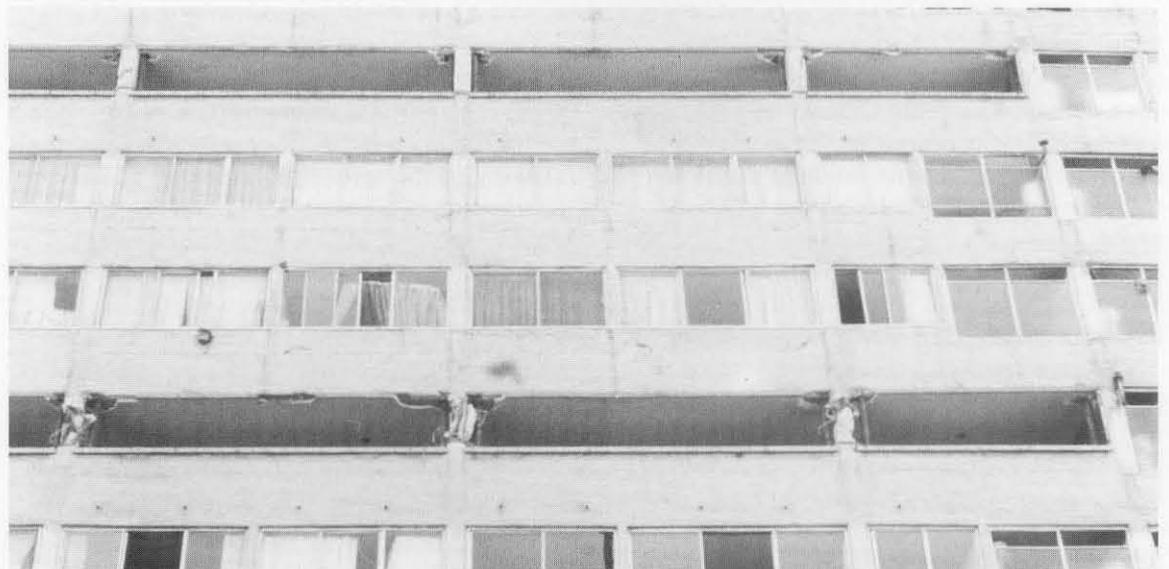
*In design, ductility is interrelated with strength because if the strength of a building is too low, then the ductility demanded by an earthquake is very high. In Mexico City, lack of strength was evident in the columns of many buildings. When such buildings survived, they did so by narrow margins.*
