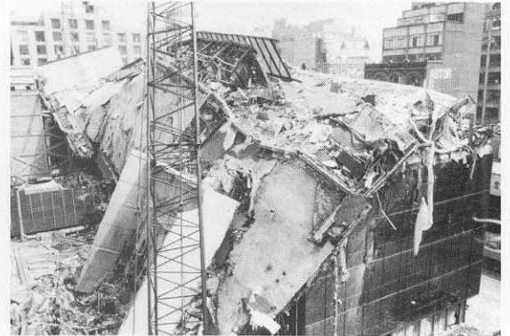
*Flat-plate construction, consisting of reinforced concrete slabs and columns without beams, did not fare well in the earthquake. Inadequate shear strength in the slab-to-column connection resulted in pancake failures of the slabs with the columns remaining upright in many cases.*
