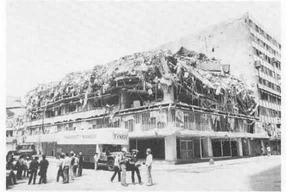
*An interesting characteristic of the damage in Mexico City is that a great number of buildings collapsed in their top stories, leaving the lower portion intact. Three examples are shown here. One possible reason for this behavior is that designers tapered the column sizes too severely in the upper stories, permissible if only gravity and wind loads act, but unwise for earthquake loads.*
