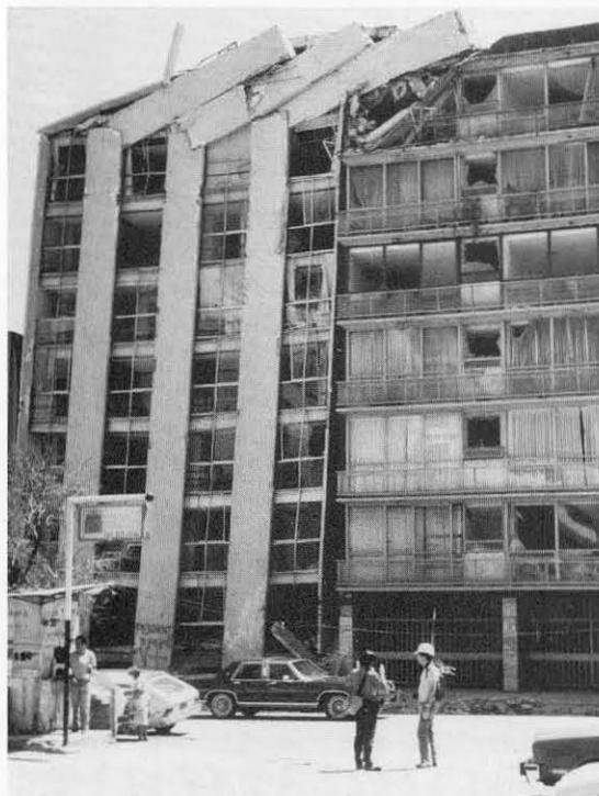
*During the earthquake, buildings swayed back and forth; a 15-story building may have swayed as much as two feet at the roof level in each direction. Closely spaced buildings thus have the opportunity to damage each other through impact. These photos show examples of impact damage; the lower one suggests another reason why the top portion of some buildings collapsed.*
