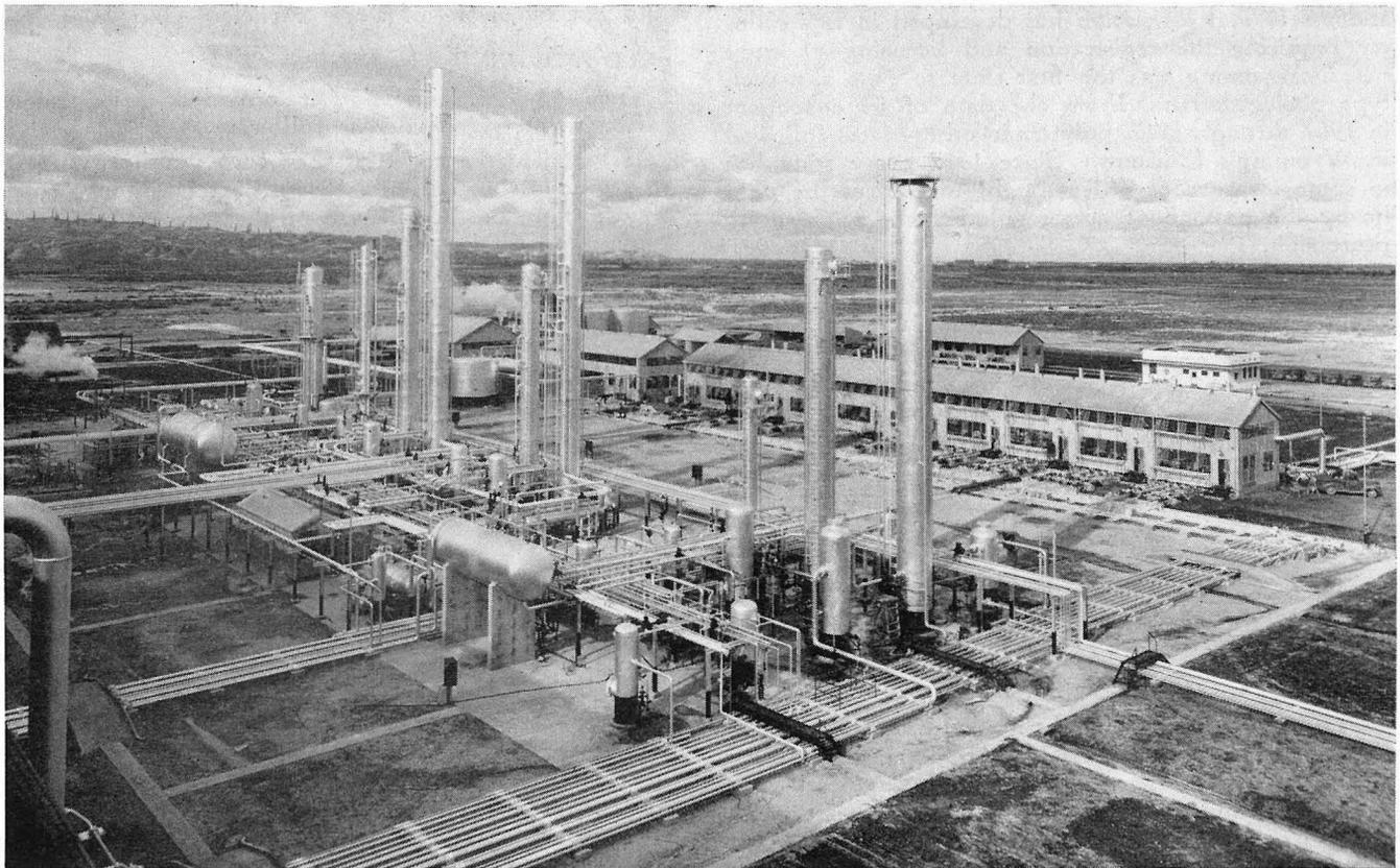
Figure 1. Modern recycling plant showing compressor building housing units which compress injection gas to 3700 lb/in.<sup>2</sup>
