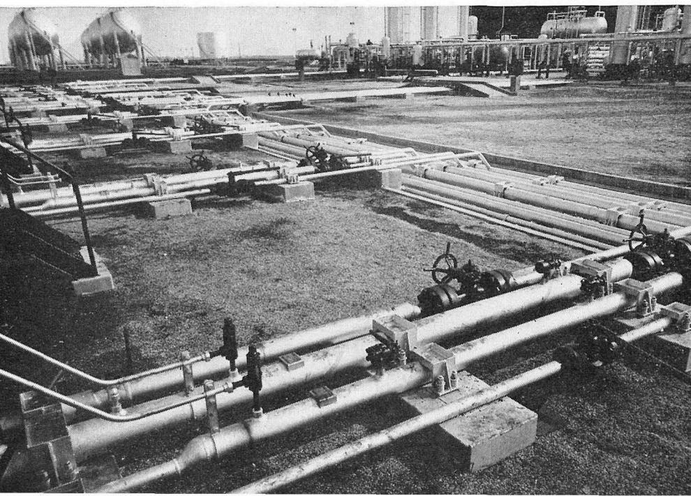
Figure 3. Pulsation dampener installation on 1500 and 3700 lb/in.<sup>2</sup> discharge laterals feeding into header system.
