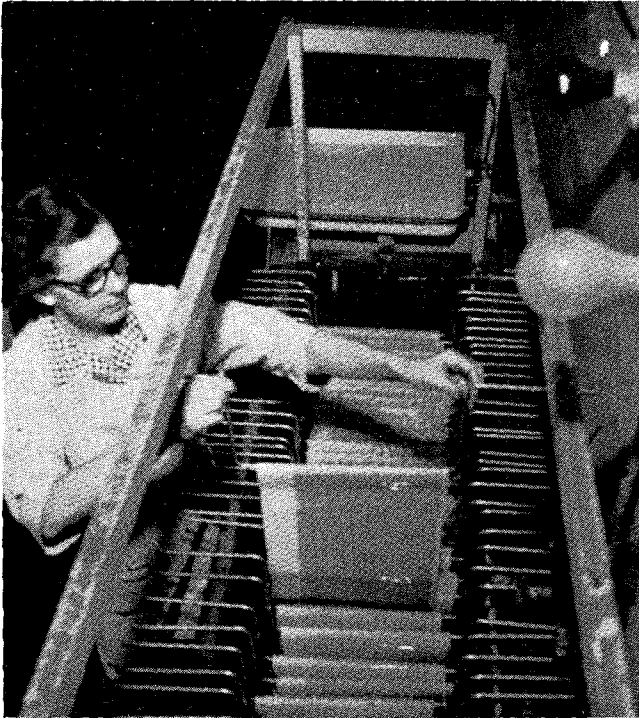
Principal recording room in the Seismo Lab has 18 photographic recorders in continuous operation. Most of these recorders are actuated by seismometers located in the tunnels bored into the hillside under the lab. They operate in complete darkness. The photo above was taken in red light. At left, girl is working on some of the 40 records which are processed at the lab every day, washing paper records. Some recorders use photographic paper, others use 35-mm. film.
