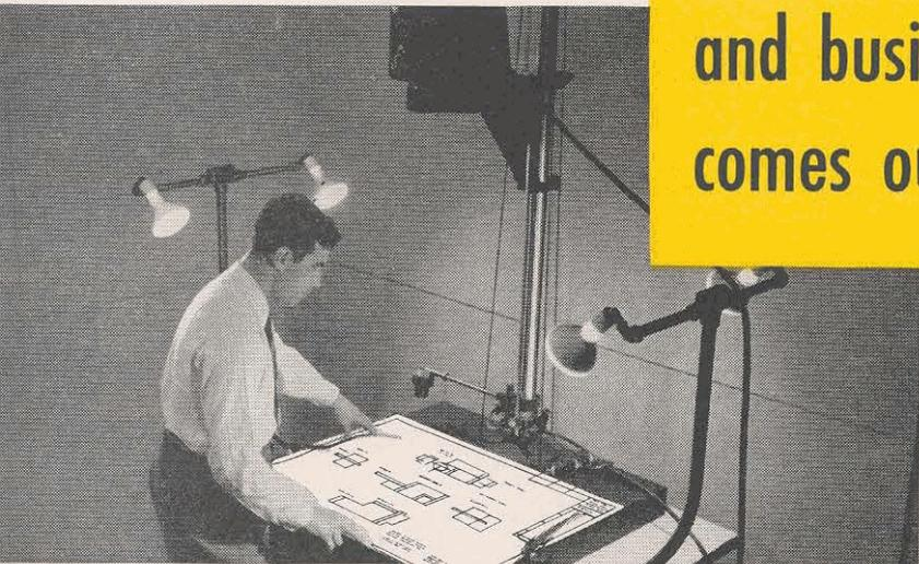
**REDUCES FILING SPACE BY 98%**—With microfilming, bulky records can be reduced and stored on a few rolls of film. 675 drawings, 24" x 36", can be recorded on a 100' roll of 35mm. Recordak or Kodagraph Micro-File Film. And everything is quickly ready for reference in the Recordak or Kodagraph Film Reader.
