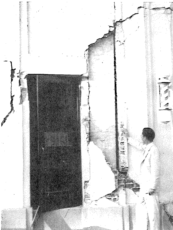
Weak brick and concrete buildings fared badly in the recent quakes. Cracks in this hotel front in Santa Barbara are the result of improper design or construction.
