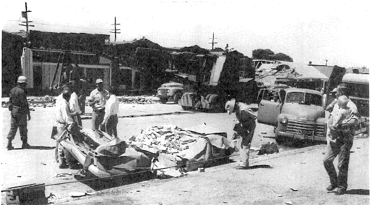
Above — all that was left of a new Ford, after the July 21 quake hit Tehachapi. An entire building front fell on it.
