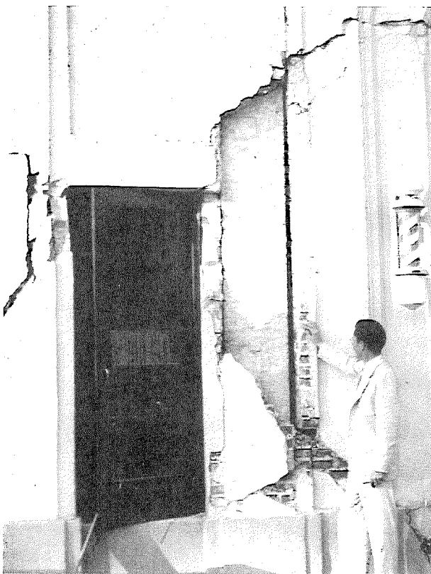
Weak brick and concrete buildings fared badly in the recent quakes. Cracks in this hotel front in Santa Barbara are the result of improper design or construction.
