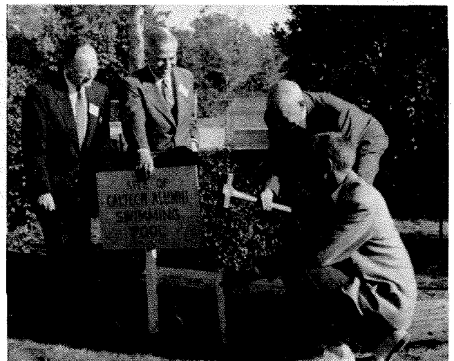
Breaking ground for the Alumni Swimming Pool
