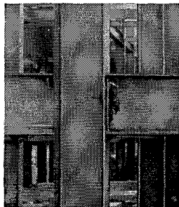
Fig. 1. Typical Riveted Connection of floor beam to column. Auxiliary steel required: 53 rivets (3/4"); 4 pieces 18" I beam; 2 pieces 6" x 4" angles; 2 pieces 4" x 3-1/2" angles.
