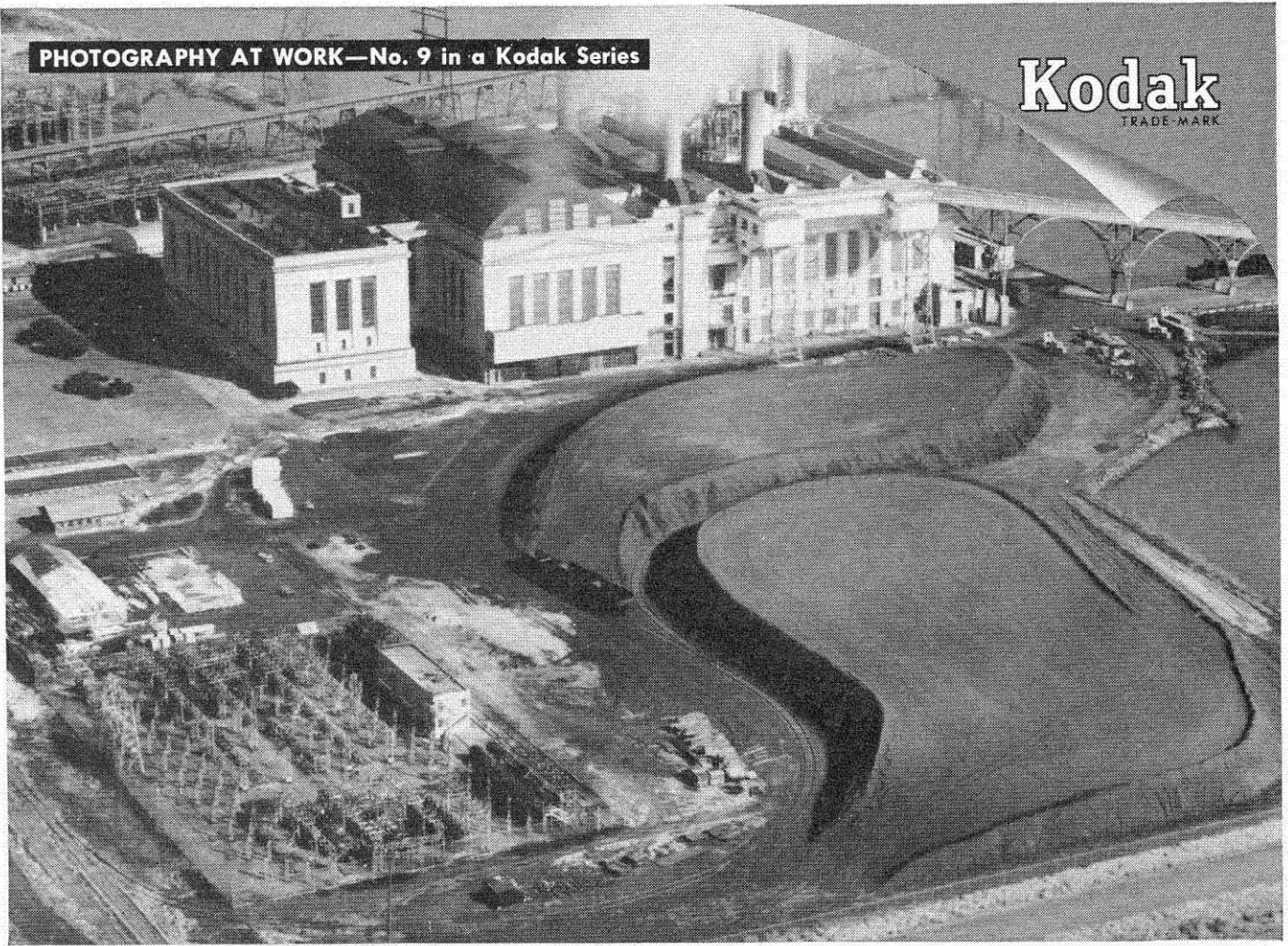
Richmond Station of the Philadelphia Electric Co.
