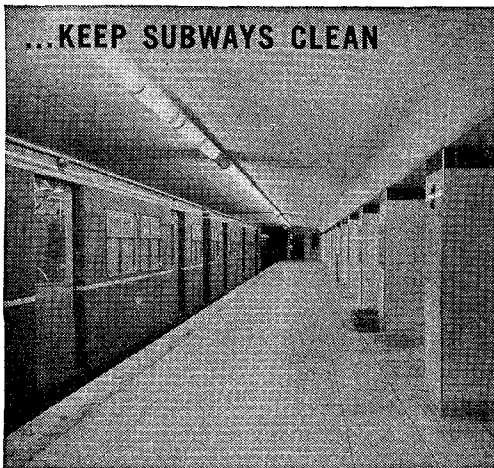
ONE PAINT IN A HUNDRED —Toronto's new $50,000,000 subway is modern in every way, including its glistening tile walls and brightly painted ceilings. For the ceiling, a paint was needed that could resist high humidity. More than 100 were tested and a paint based on Hercules Parlon® (chlorinated rubber) selected. On all types of surfaces, interior and exterior, Parlon paints are providing outstanding service at lower long-term cost.
