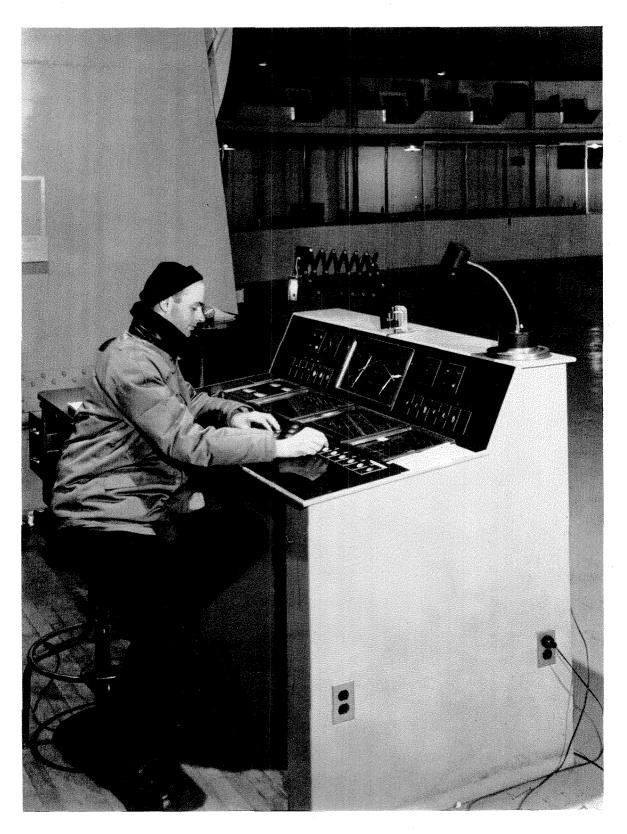
At the main control board, the night assistant sets the dials and, with a push of a button, the huge telescope moves into position. Automatically the dome turns to keep its slot in front of the telescope, open to the observer's field of study. Although the Hale weighs 530 tons, a tiny one-twelfth-horsepower motor makes it follow a star.
