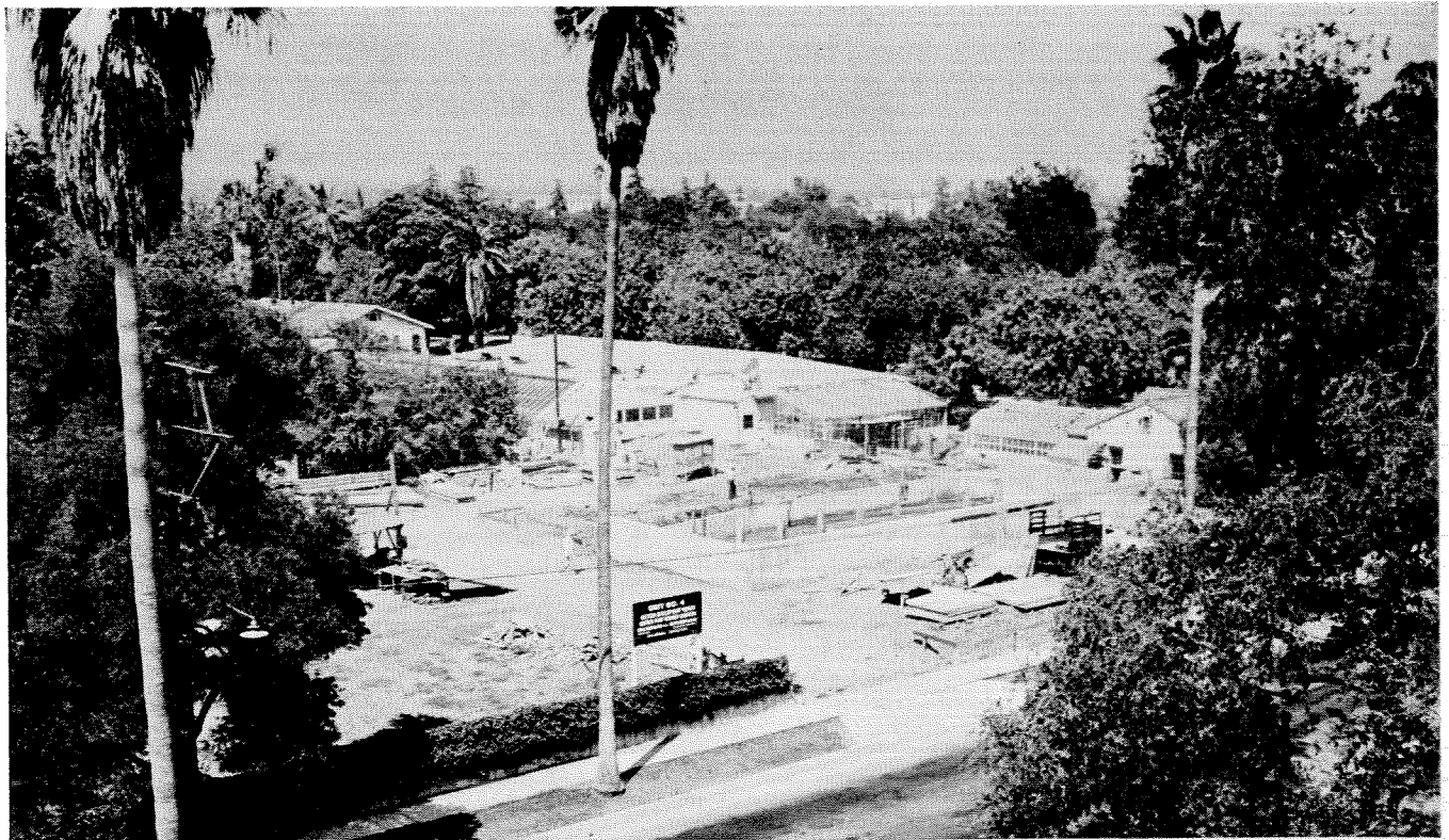
Unit No. 4, the Campbell Plant Research Laboratory, is an addition to the Dolk and Earhart Laboratories. It will provide 3,000 square feet of de-smogged, air-conditioned plant-growing space for studies of plant viruses and plant development problems.
