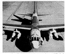
Boeing B-52H shown carrying mockups of Skybolt air-launch ballistie missiles. B-52s are also jet-fast platforms for Hound Dog guided missiles, and in addition carry regular load of gravity bombs.
