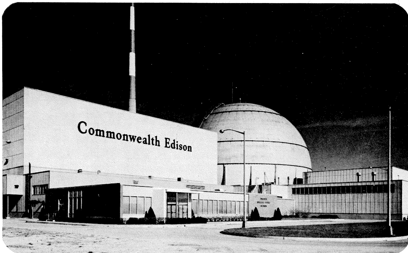
DRESDEN NUCLEAR POWER STATION —America's first full-scale producer of commercial electric power from the atom, rated 200,000 kw.
