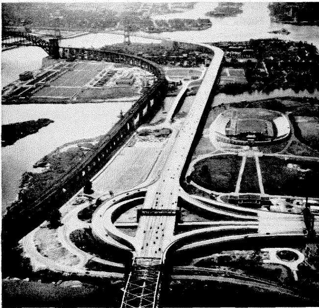
Randalls Island, N. Y., Traffic Circle Triborough Bridge in Background
