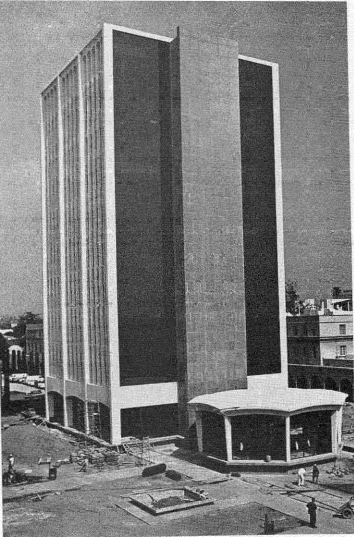
The new library in the final stage of construction.
