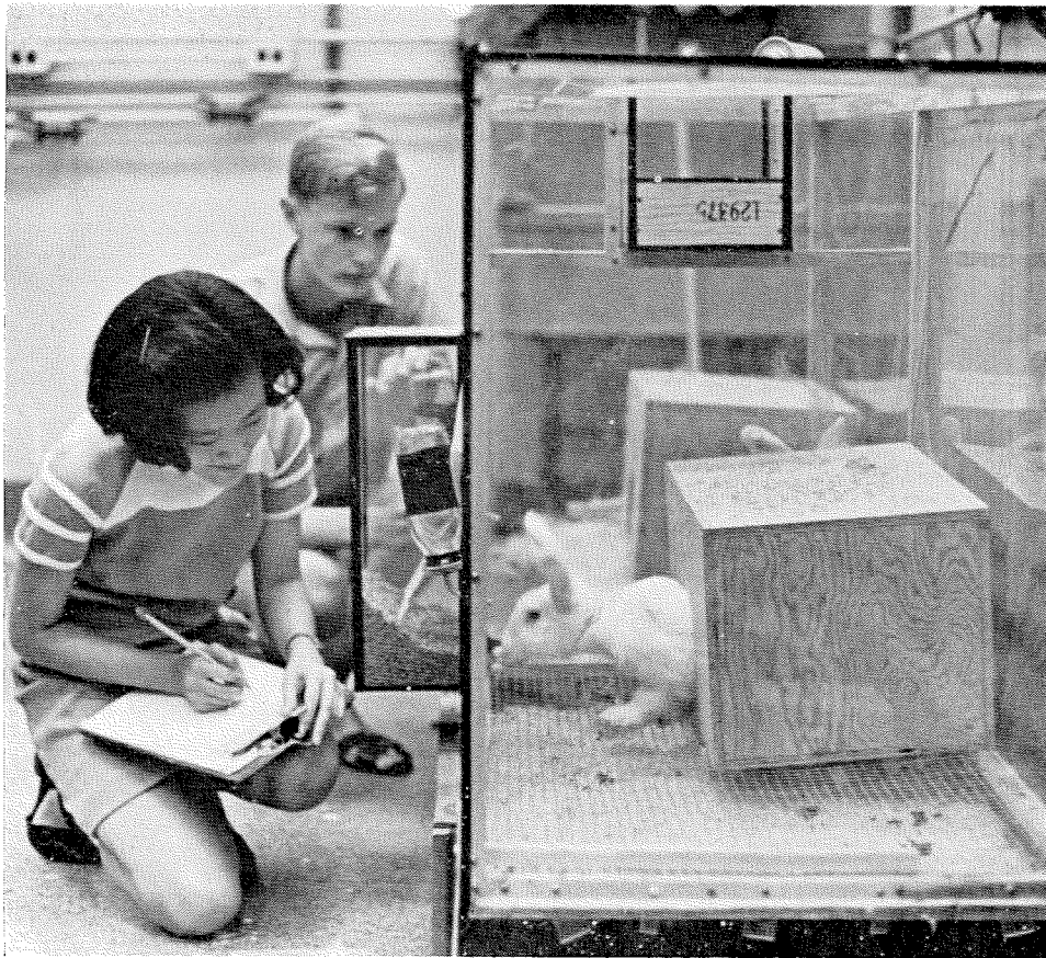
Project workers compare blood samples of rabbits in smog-free and smog-filled chambers. Results show that rabbits breathing smog have 25 percent more lead in their blood.
