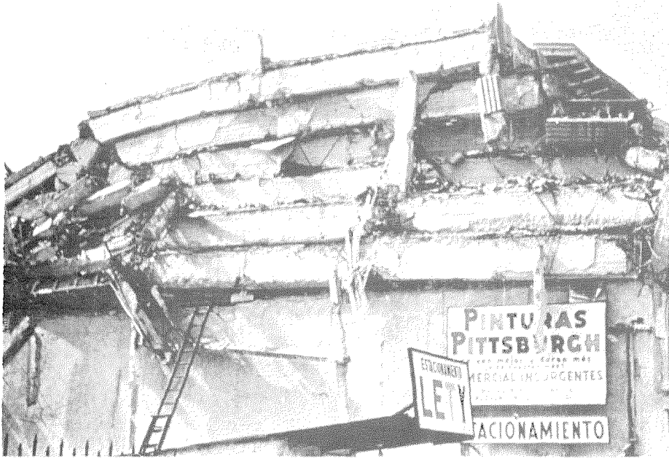
This eight-story building in Mexico City telescoped into a pyramid-shaped structure as a result of the 1957 earthquake.
