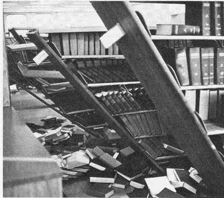
Nearly all the bookshelves collapsed on the upper stories of Caltech's Millikan Library, and about 75,000 books spilled to the floor. The accelerograph at the base of the library recorded a maximum acceleration of 15 percent g, and the instrument at the top of the building showed about 35 percent g.
