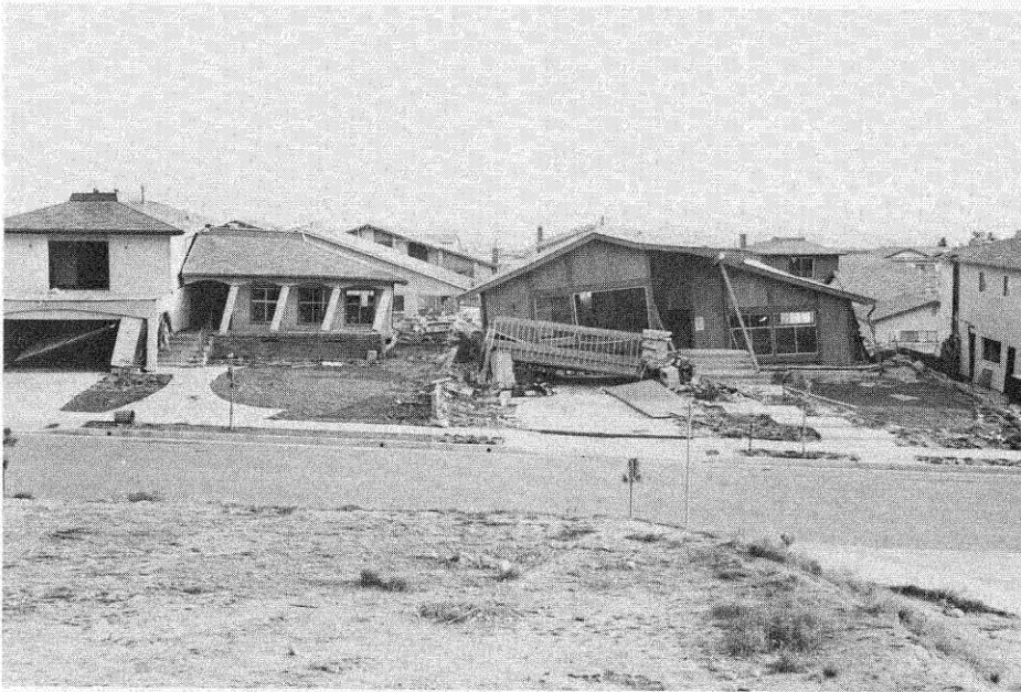
Modern residences of “non-typical” design and construction suffered heavy damage in the San Fernando earthquake. These split-level homes near Sylmar did not survive the strong ground shaking.
