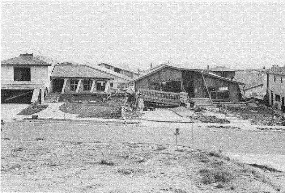
Modern residences of “non-typical” design and construction suffered heavy damage in the San Fernando earthquake. These split-level homes near Sylmar did not survive the strong ground shaking.
