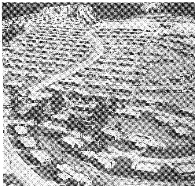
Workers' homes at Los Alamos atomic weapons plant.
