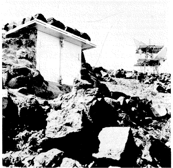
A Caltech telemetered seismometer vault, with an AT&T microwave repeater station in the background, at station GLAMIS, near the California-Arizona border north of Yuma.
