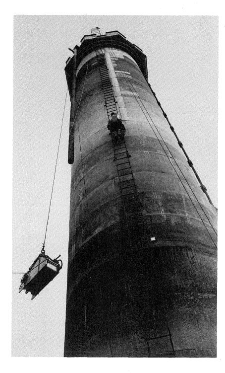
A Housner-Hudson shaking machine, the first modern earthguake-simulation device, is hoisted to the top of a 110-foot intake tower at the Encino reservoir in the San Fernando Valley for the first field test of the machine in 1961. Although this tower was scheduled for replacement and could be shaken with the energy equivalent to a fairly strong earthquake, a similar machine on Millikan Library jolts that structure only gently for student projects.
