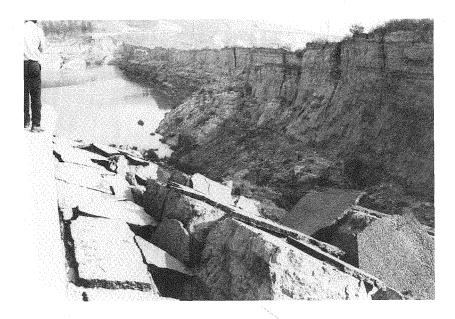
Dams hold a great potential for destruction and loss of life in an earthquake. Although a large section of the Van Norman dam (built in 1916) failed and slid into the reservoir during the 1971 San Fernando earthquake, the dam itself survived. This was not part of the Feather River project, whose earthquake engineering standards, developed by Housner, set a precedent eventually adopted worldwide.
