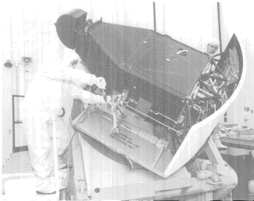
**Technicians put the final touches on the Wide-Field/Planetary Camera.**
