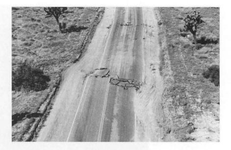
**Right: This asphalt** road near Landers exhibited one of the first offsets observed by the helicopterborne geologists. **Below: Another fence** offers a clear illustration of right-lateral slip, in which objects on the far side of the fault appear to have been shifted to the right. The fault runs horizontally through the middle of the picture.
