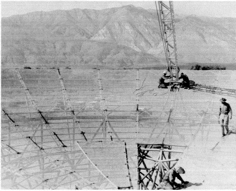
**The reflectors (far left) were made of steel mesh with 1-cm holes. The 45-foot pedestals, or towers (below), were constructed separately and the dishes hoisted onto them later.**
