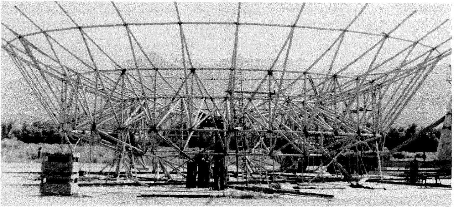
**Above: The skeleton of one of the 90-foot dishes rises against the Sierra Nevada, which borders the valley on the west. Below: Workers position the hub at the center of the dish.**
