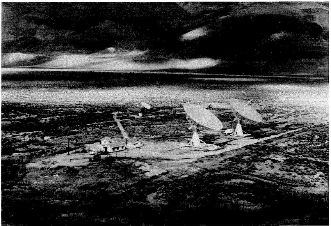
**Right: OVRO from the air before the north arm was begun, probably in 1959. The living quarters and the shop are visible in the foreground and the 32-foot dish just above it. Between the 90-foot dishes, behind them, the low-frequency array of dipoles is also faintly visible. Below: Workers construct the tracks of the east arm in 1957.**
