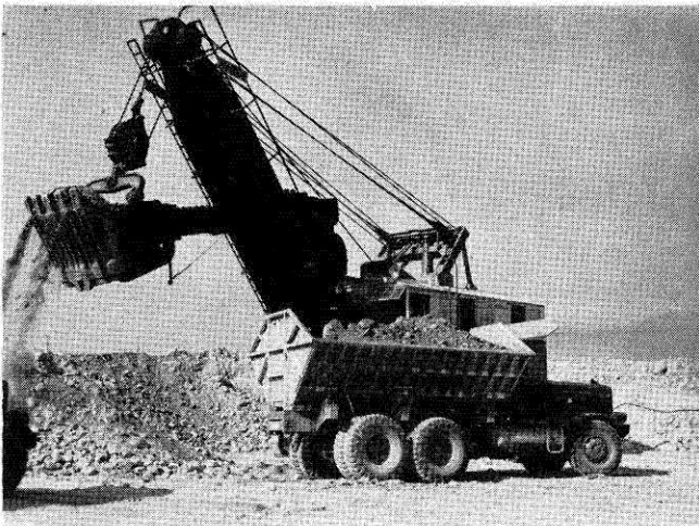
Loading a 25-cubic-yard side dump truck with a six-cubic-yard electric shovel.
