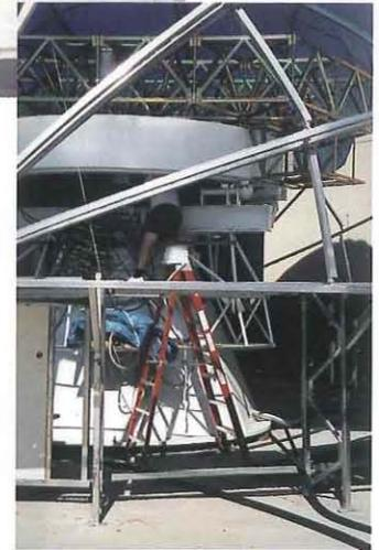
(see *E&S*, 1996, No. 4) is taking shape (right). (That's Steve Padin, chief scientist for the Cosmic Background Imager, on the ladder.) The framework (above) will support 13 one-meter radio telescopes. Assembly and testing will continue through August or so, after which it will be dismantled and
