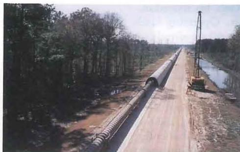
As seen from inside (above), a beam tube, at four feet in diameter, is almost big enough to stand in, hunched over. The tubes are laid out in sections on a concrete slab (right) and then covered with sections of concrete arch, six inches thick, seen here partially finished at the Louisiana site. The completed tunnel, in the less verdant expanse of Washington (above right), has access entrances every 250 meters.
