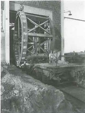
Left: The prime focus cage was so large that the Westinghouse factory door had to be enlarged and the track lowered four feet to get it out.
