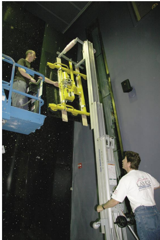
The upper panels were installed using a lift equipped with those suction cups you normally see in bank-heist movies when a plate-glass window needs to be cut.
