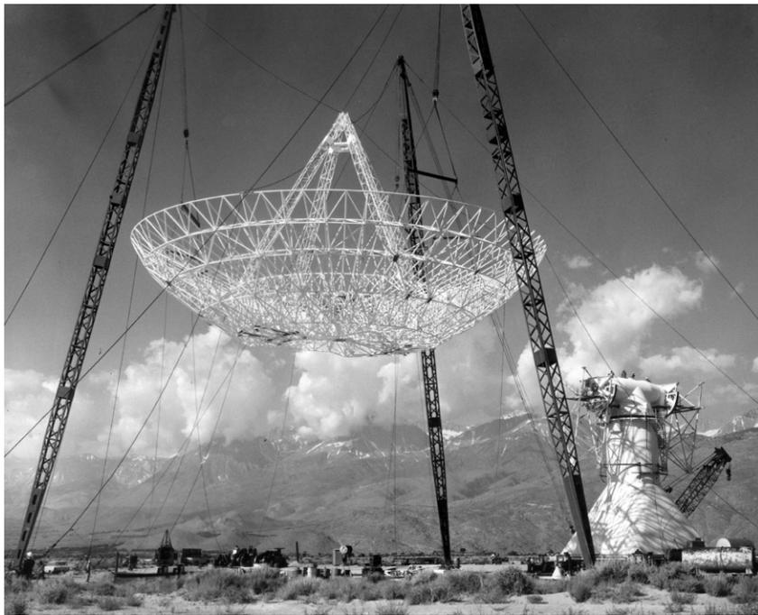
**The 40-meter radio telescope dish being lifted onto its pedestal in July 1967. Once the dish is high enough, the base, which has already been mounted onto its railroad tracks, will be driven into place underneath it.**
