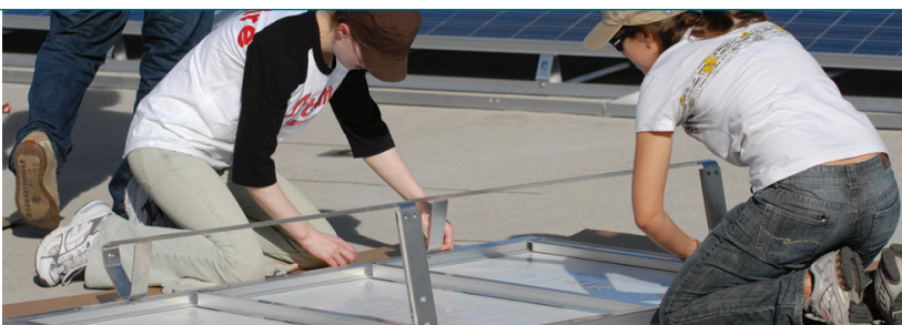
Atwater postdocs Dierdre O'Carroll and Marina Leite install the support structure on the back of a solar panel.
